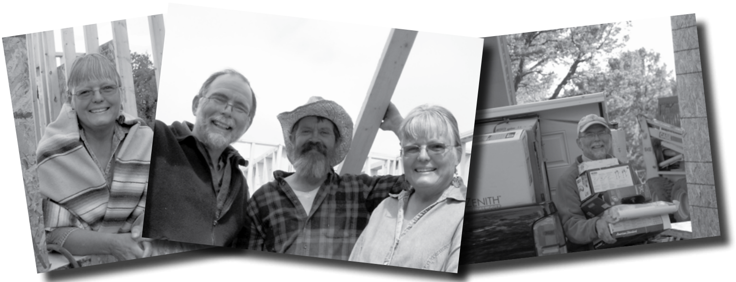
Tessa, Fr. Dave, and contractor Denny Ertle enjoy the early stages of building Tessa's new hermitage.
